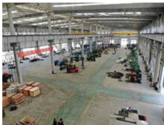
Kaiyuan Production Facilities
